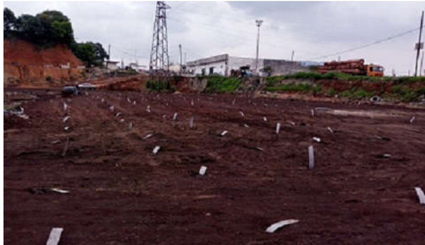
Figure 3 Some vertical drains put in place
